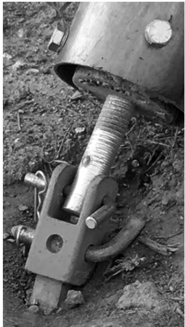
INCORRECT Brace-to-HGA Connection
